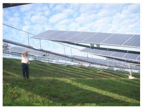
**Figure 1:** 650kW Solar Wings Plant at Lonza Solar Park in Waldshut, Germany. Polycrystalline Silicon modules (230Wp) are mounted in groups of 8 modules on of the 310m long mounting and tracking cable. 6 standard AC motors powering the standard linear drive to move the one axis tracking cables.
