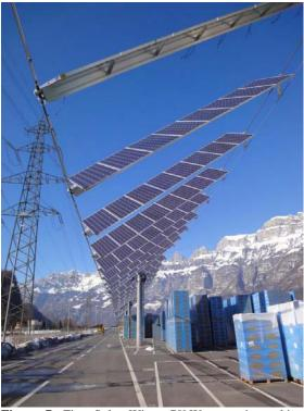
**Figure 7:** First Solar Wings 70kW two-axis tracking system installed at the Flumroc AG, Flums Switzerland and in operation since spring 2010.
