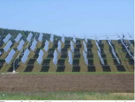
Figure 2: Solar Wings tracking system at the Lonza Solar Park with a mounting distance of the WINGS of about 5m.
