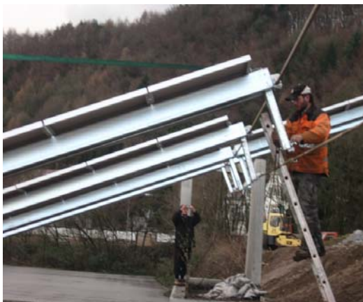
Figure 2: Beams are connected to the tracking cables.
