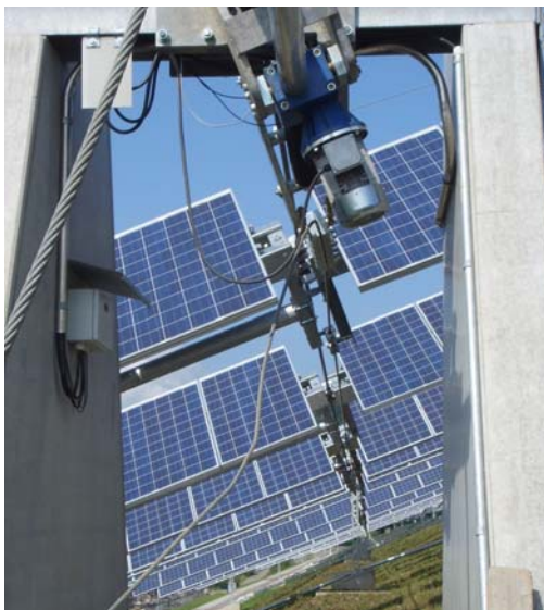
Figure 3: Solar Wings tracking system showing a view along the 310m long tracking cable, with the standard AC motor powering the standard linear drive to move the tracking cable (Lonza Solar Park).
